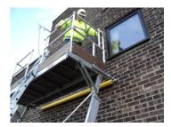
Climb onto the Platform and position the rear Uprights into the rear locating sockets on the Platform for both the Left and Right handed Guardrail. Make sure all uprights have been secured with Pins & 'R' Clips provided.
