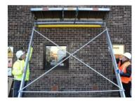
With bent Legs and a straight back, lift the Solar Platform firstly to waist height, then using your arms to offer it to the wall and roll it up into position.
