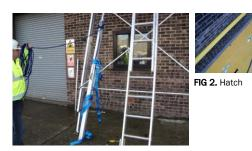
Close the Draw Bar before hoisting the Hoisting Assembly to the platform. NOTE: The Hoist Assembly should always be lifted through the Solar Platform Hatch.
