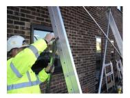
Remove top  $\operatorname{Pin}$  and fit to the Back Leg at about eye level to the Main Leg.
