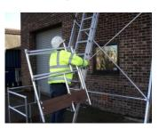
Position the Right Guardrail over your shoulder, when climbing the Ladder, maintain three points of contact. REMEMBER: When fitting the Guardrail to the Left hand side of the Platform carry up on the Left shoulder.
