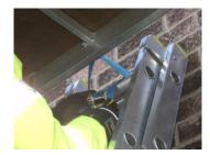
Secure the Platforms to a solid substrate, ensuring the wall tie Is securely fixed. Consult a fixing specialist if unsure.
