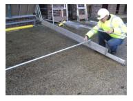
Fit the Horizontal Cross Brace over the retaining studs.
