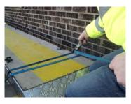
Using the 2 'Ratchet' Straps provided, fix the 'Catwalk' to the Platforms as shown above. Pass the straps round the 'Horns' of the Platforms frame and Catwalk, tightening the buckle in a position where it will not trip the user. NOTE: Always ensure the Catwalk is free from obstructing the Solar Platform Hatch.
