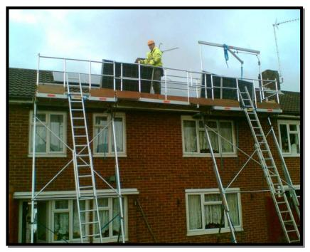
Temporary access device conforming to the test requirements of BS EN 12811 CLASS 2 & EN 13374 CLASS C
