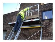
Feed one arm through the top rung of the Ladder this provides a handhold when offering the Guardrail into position. (NOTE: This is why the Ladder needs to be extended above the platform by 1 metre to provide a handhold)
