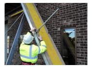
Stand the Catwalk up against the Platform and Install the Centre Uprights on the Catwalk and secure with Pin and 'R' Clips. This will allow assembly of the Guardrail Set prior to access.
