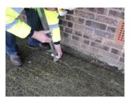
Drop the feet to the ground and take it up to the next hole and secure with the Pin and 'R' Clip. Ideally a finger's clearance under them to ensure the Solar Platform remains in contact with the wall.
