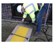
Tie a rope through the end Guardrail sockets and secure.
