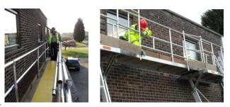
Fit the inner Guardrail the same way as in STEP 27. Remember to be clipped on with a lanyard at all times when fitting the Guardrails whenever possible. Secure all Toe Boards to the Uprights.
