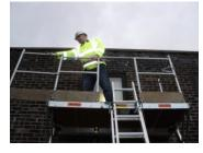
In order to prepare the Platforms to receive the Catwalks, clip on with a Lanyard and remove the Pin and 'R' Clips from the Internal end Guardrails and fold them outwardly. Repeat for the second Platform. This will provide access for the Catwalk to be positioned. Repeat **STEPS 1-20** for the assembly of the second Platform.
