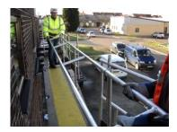
Whilst still clipped on fit the end Uprights and position the front Mid-rail and Top-rail over the Uprights from the 2m Platforms. Tighten all grub screws and secure Uprights with Pin's and 'R' Clip's provided.
