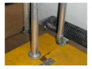
Attach the support frames at both ends to the retaining sockets ensuring the flange is clear of the hatch and flush with the Platform.
