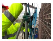
Lift the whole assembly by holding the support tubes and then position these tubes over the Holes in the end support frames. **NOTE: Two operatives are required to complete this assembly.**
