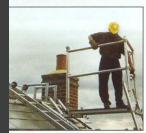
Fit handrail and engage interlock clips.
