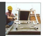
Release the support frame and swing out towards the eves of the roof. Engage the hooks so that the frame is angled towards the eves and not under the platform.
