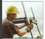
Level the platform and engage the cross pins.
